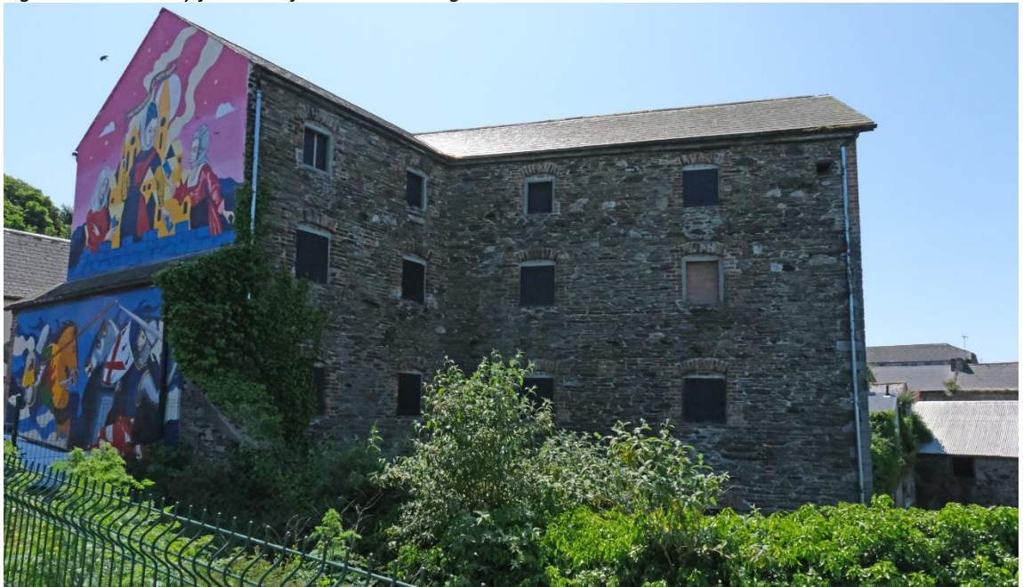
Fig.14: View of the grain store from the north showing the north gable and off-set return.
