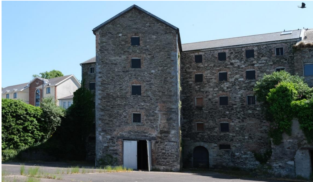
Fig.16: The rear (west) elevation of the grain store, with hard landscaped courtyard.
